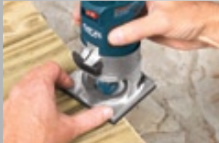
Round Off Deck Planks & Rails
